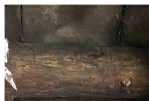
Log beam discovered in the rear wing of the Evans house. Photo by Carol Lasser.
