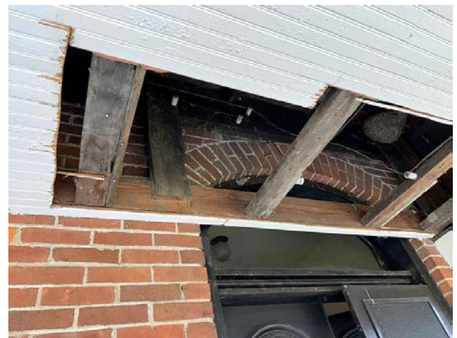
Front entrance of the Evans house with a portion of the 1927 porch ceiling removed to show evidence of an earlier porch roof and arched header over transom window. Photo courtesy of Naylor Wellman..
