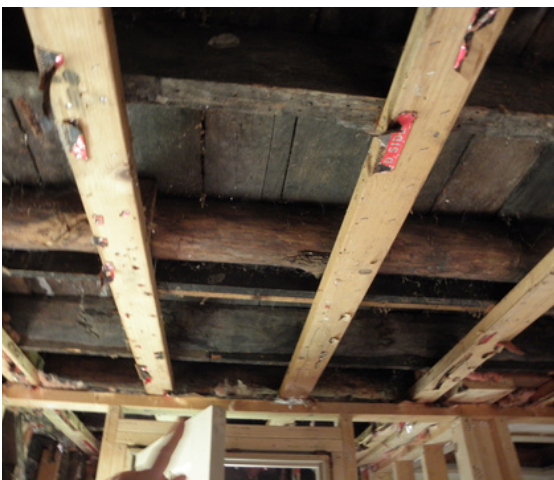
Log support of loft over the rear of the kitchen wing. Photo by Karen Schaefer.
